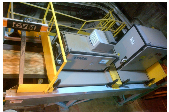
Figure 1: CMS installation at Zellstoff-Celgar ahead of the chip bin
